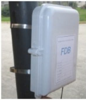
FDB fiber termination box on the pole
