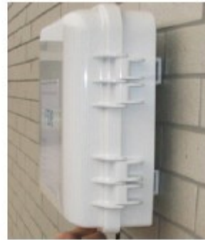
FDB fiber termination box on the wall
